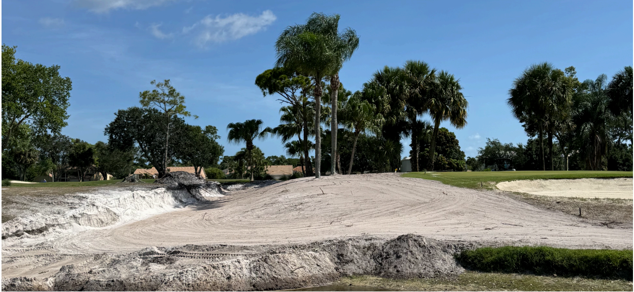
#8 Green surround, Bunker, Lake Bank, and Irrigation project began in June.
