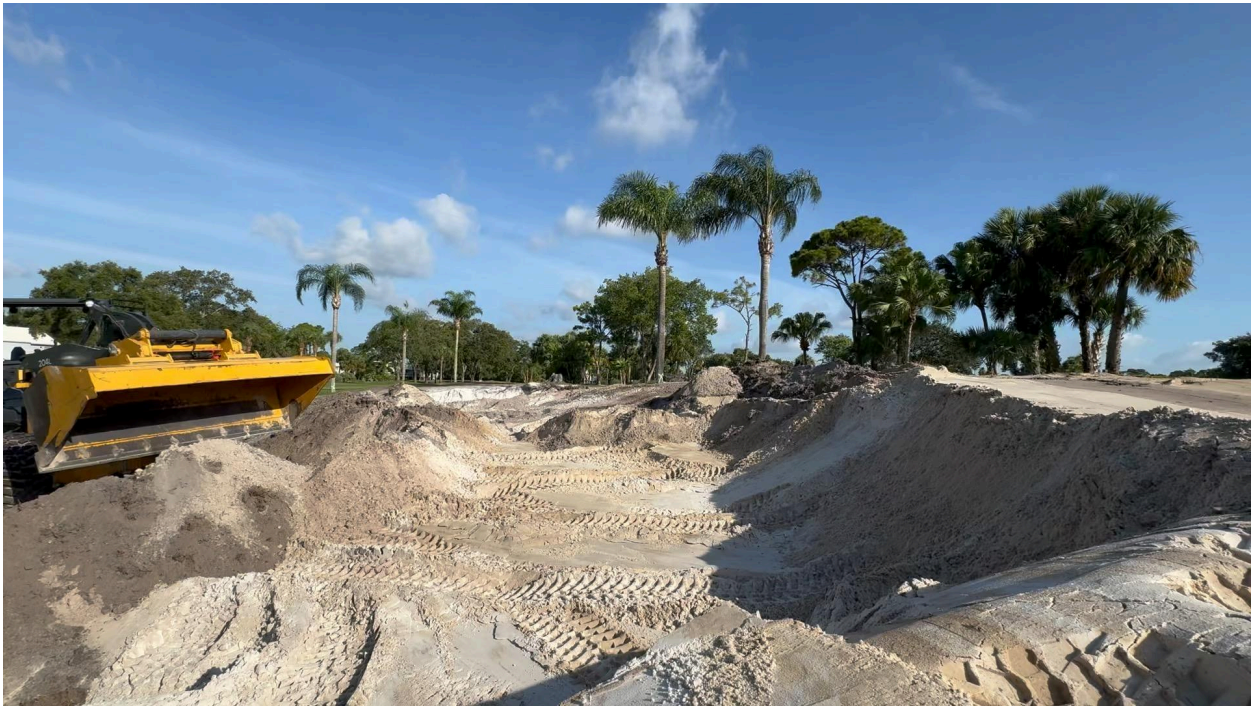
#8 Green and Bunker construction.
