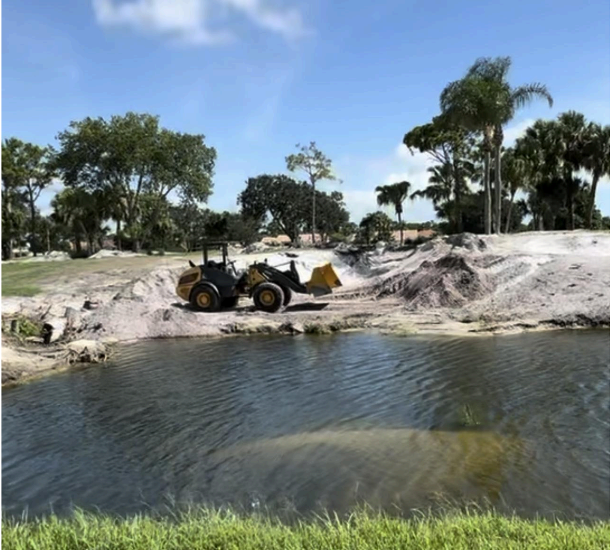
#10. Relocating soil from project area to Green Surround on #8.
